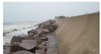
**Dikes:** Shore-parallel features, often built of unconsolidated material, mainly to address the flooding hazard in low lying areas. They might be combined with harder protection structures such as revetments to prevent erosion.
